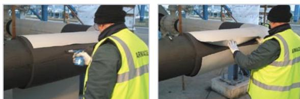
1. Apply a minimum 50 mm glue line with the correct type of Armaflex adhesive to the surface of the Armaflex and the underside of the Arma-Chek S+ covering. Correctly position the covering along this line and, when satisfied, apply firm pressure. Smooth the covering around the circumference for a clean finish.
