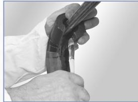
6. Cut the fitting piece open along the inside "throat". Install the fitting piece on the pipe. Apply the appropriate Armaflex adhesive on the "throat"-seam.
