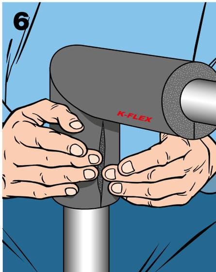
**INSULATING AN ELBOW with tubing of different diameters**
