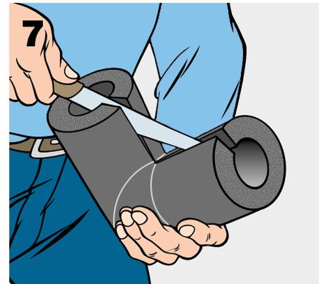
Slide the elbow section over the pipe and carefully glue the edges together.
