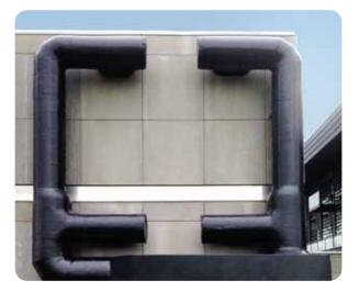
An overlap of only 20 mm is sufficent in order to provide protection to the insulation and duct system itself.
